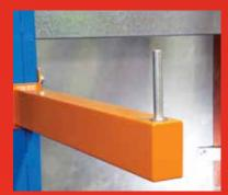
Turnbuckle bracing provides lateral stability. It also allows for re-adjustment of the structure if required.
