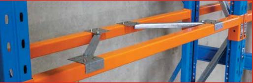
Plan bracing is used to brace the structure across the horizontal plane.
